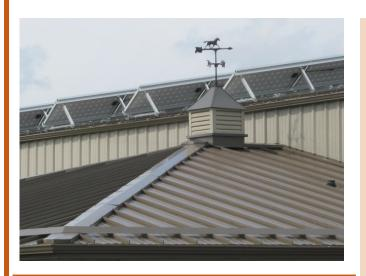
\*Oil Canning: Flat metal surfaces can display waviness, commonly referred to as "oil canning", which is an inherent characteristic of steel. "Oil canning" is not a defect and therefore not an acceptable reason for rejection.
